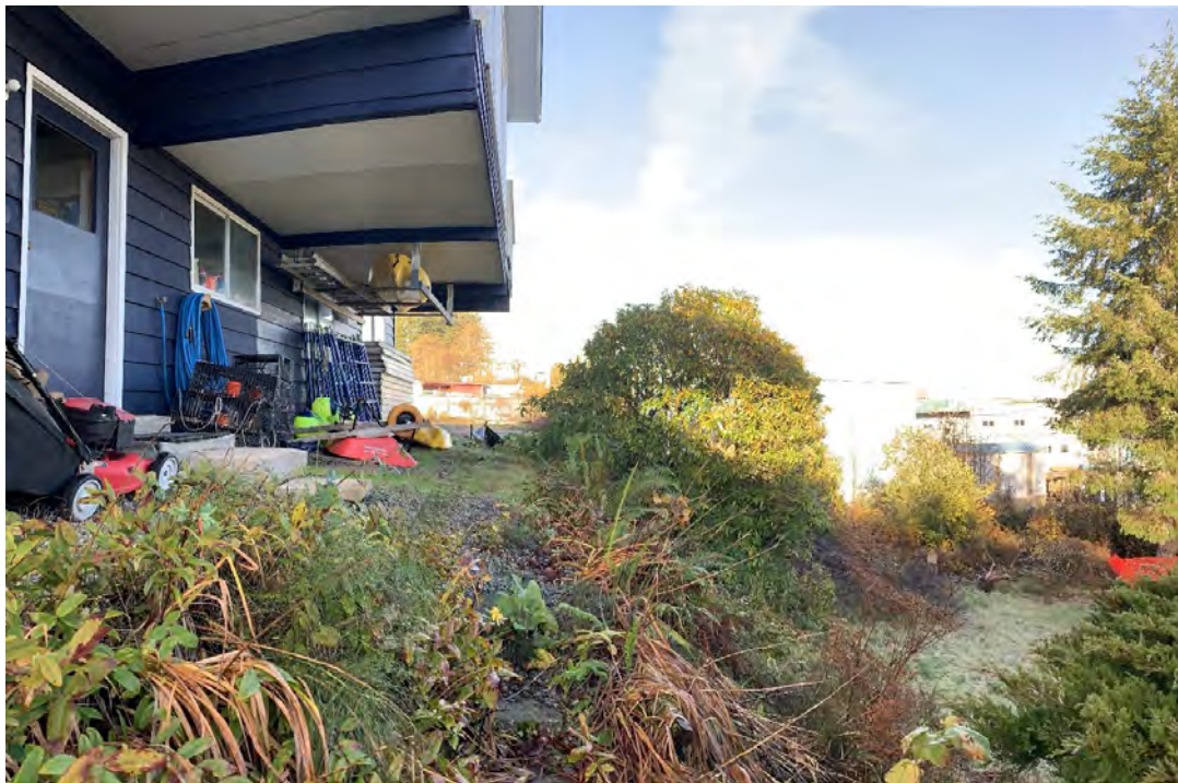
Photo 5. Photo of 1567 Imperial Lane showing the north side of the residence and the backyard, (November 16, 2023)
