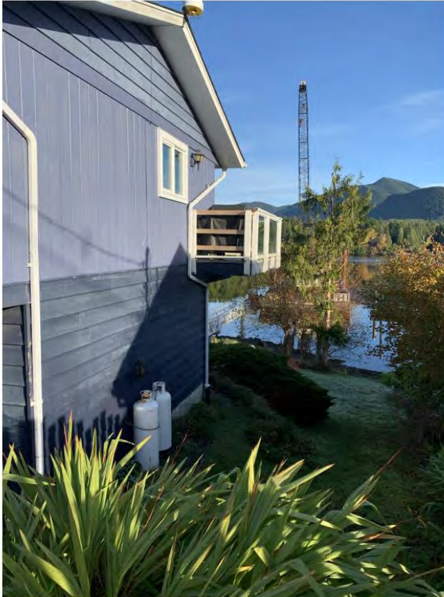
Photo 3. Photo of 1567 Imperial Lane showing the east side of the residence. (November 16, 2023)
