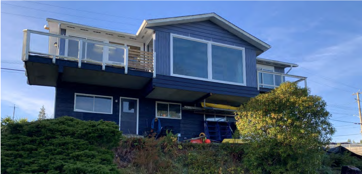
Photo 1. A photo of the back (north) of the house at 1567 Imperial Lane, with the existing deck.
